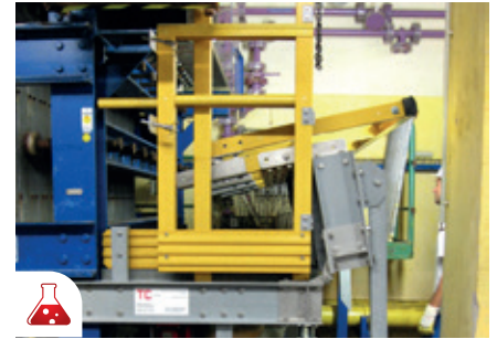
Foldable GRP platform for a chemical plant
